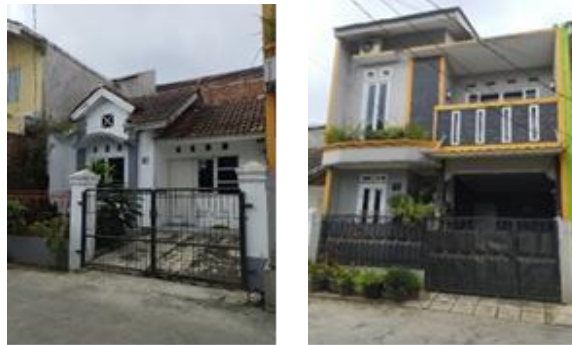
Figure 13. Left before renovation, right after renovation
