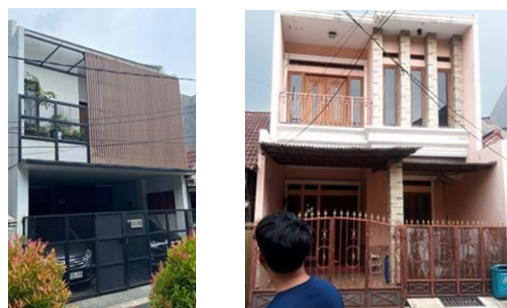
Figure 6. House after renovation
